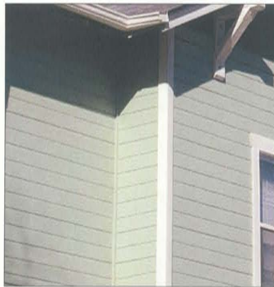
Painted horizontal wood siding
