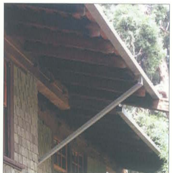
Large overhangs and exposed rafters
