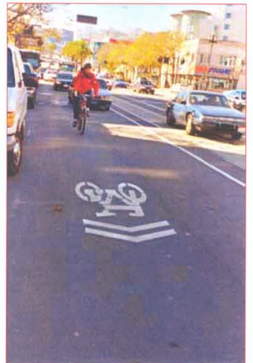
Right: Examples of 'Sharrow' types of streets where cyclists and motorists share a narrow and calm street.
