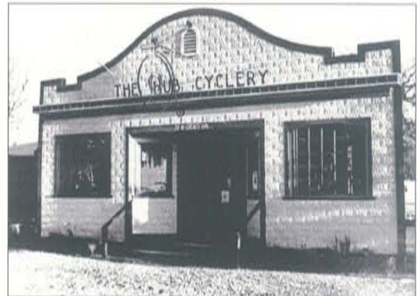
C. Frengle Metal Shop c. 1930, also The Hub Cyclery in 1990's
