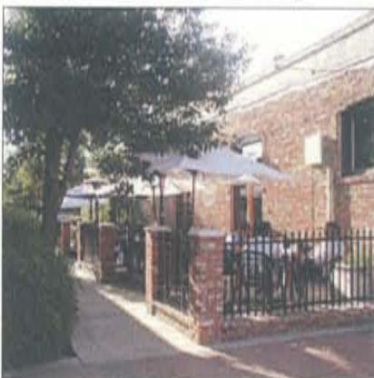
Liner building transitioning to sidewalk
