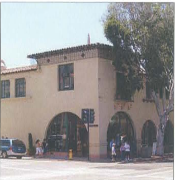
Vertical articulation of corner
