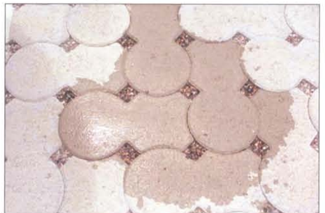
Pervious paving to minimize flow across pavement
