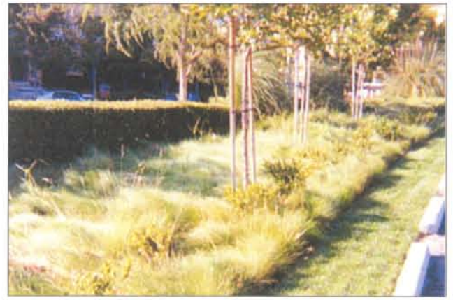
Stormwater drainage directed to bioswale
