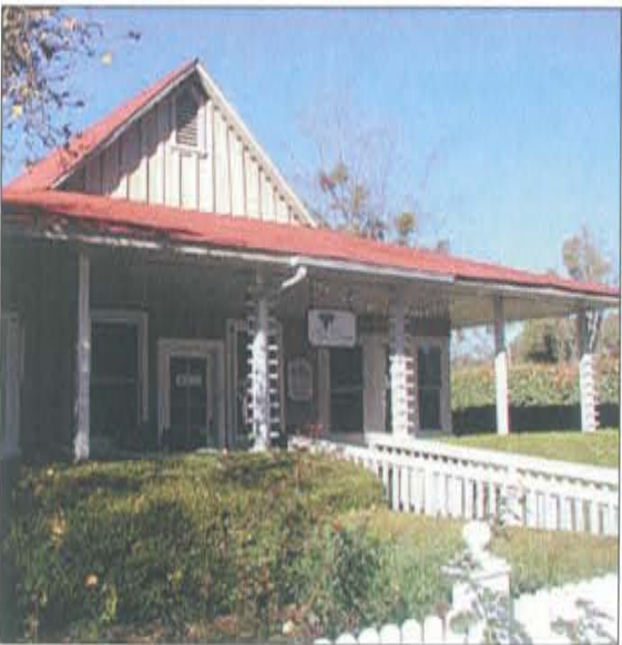
Composition shingle roof
