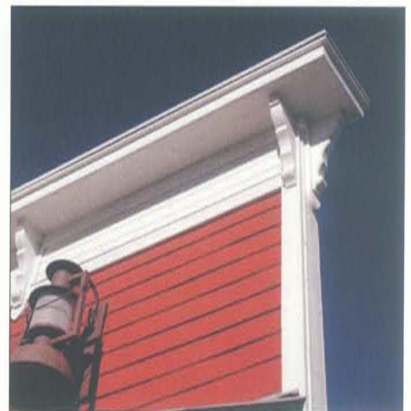
Parapet with cornice and brackets
