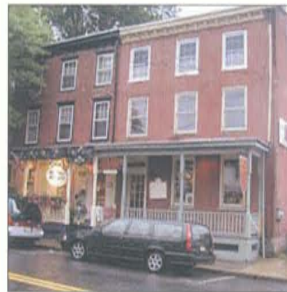
Above: 3 story mixed-use building
