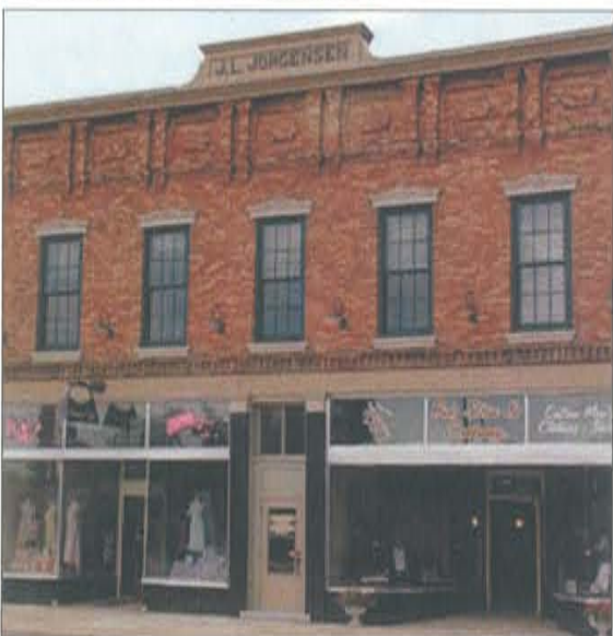
Articulated parapet denotes center, entry
