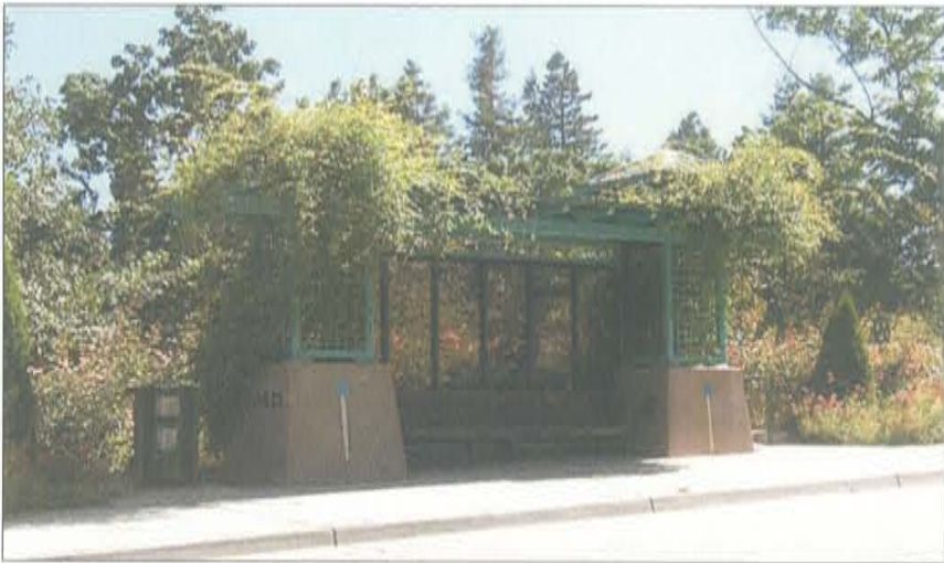
Above: Sonoma County Transit Stop on West Sierra Avenue
