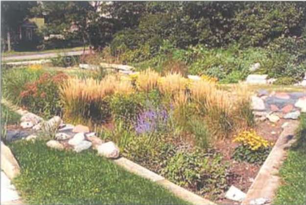
Rain garden to capture roof run-off
