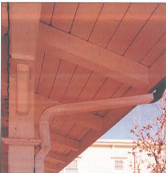
Gutter and downspout
