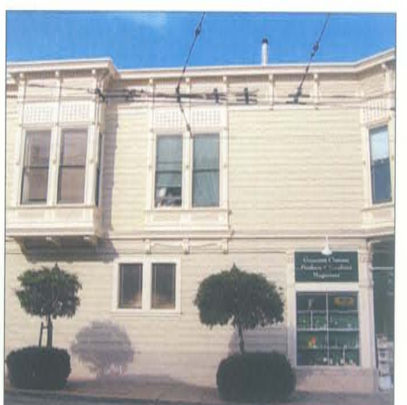
Projecting bay windows
